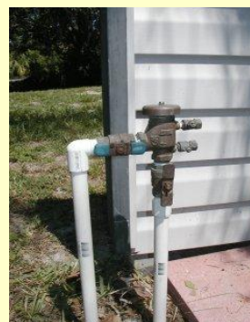
Common types of backflow preventer
